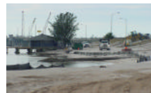
Ringling Causeway Project
